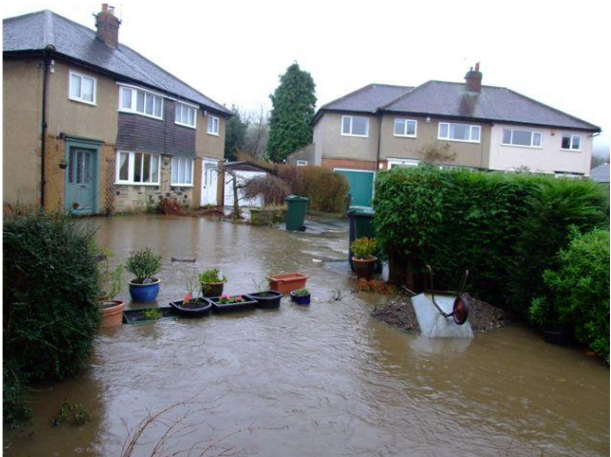
Flooding at Moorfield Avenue
